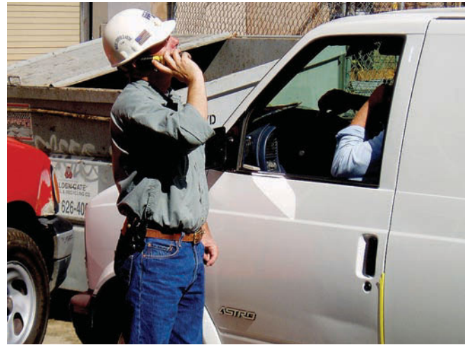
An independent contractor communicates from a building site. What are some significant differences between employees and independent contractors? (Greg Younger/Creative Commons)
